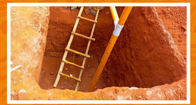
Step 2: Excavate for soak pit approx. 7ft long by 6ft wide and a depth of 7ft
