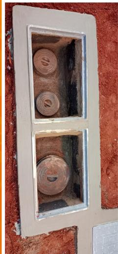
Step 7: Make provision for 2 inspection points/ manhole covers -600mm by 450mm as shown in the picture
